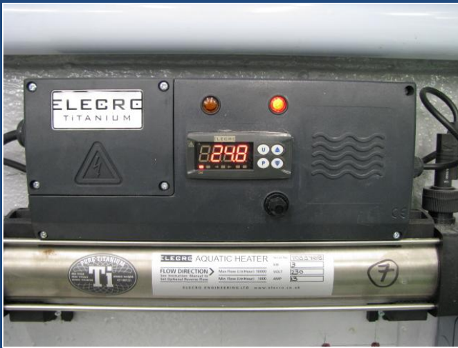
3 kilowatt external heaters
